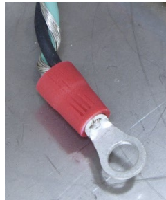
Figure 2-53: Ground Wire Termination
